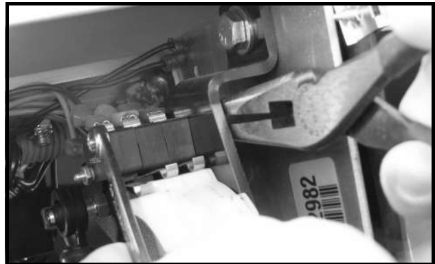
Figure 14-19 Removal of Limit Switches
